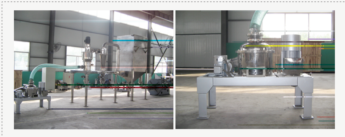
(Operation of the equipment at site)
